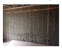
**Rock** *Wool* Filled Wall Cavity Fully Protecting Plumbing and Electrical
